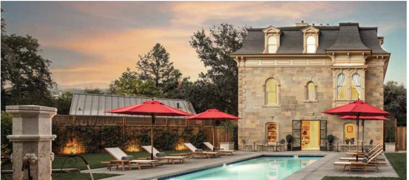
Top, back of the house at The Francis House. Bottom, interiors of the remodeled Francis House [Photo by Michael Hospelt]
